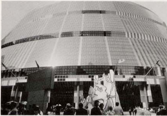
State of Illinois Center (4)
